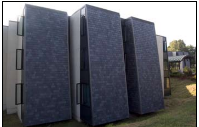
The dormitories feature unique mansard roofs that reach from the top of the buildings down more than four stories to the lawn below. DaVinci Slate was selected for its durability and style to the vertical applications of the buildings.
