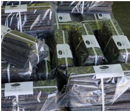
Bundles are delivered custom shaped and numbered by row.
