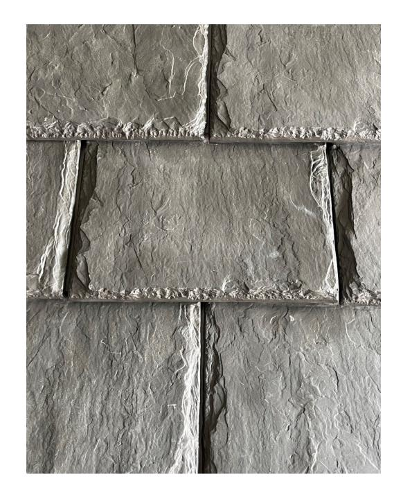
Raise the butt end of the tile that is going to be replaced. Place a flat bar under the tile to be removed and loosen 2-4 nails along the top of the same tile.
