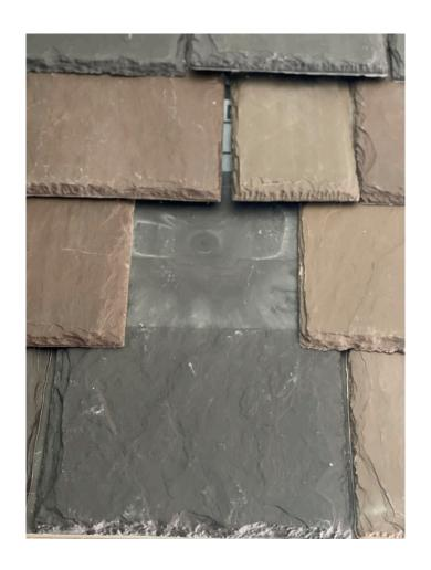
Patch any holes in the underlayment as required per the individual manufacturer and local building code. Locate a new tile of appropriate size and color that matches or resembles the removed tile and slide it into the previously occupied space.
