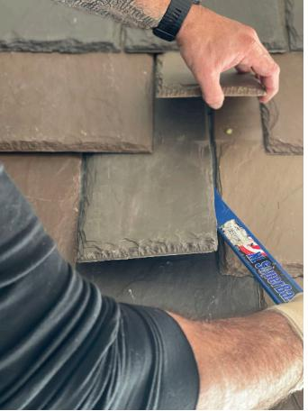
Locate fasteners in the tiles in the course above that penetrate the tile that you are replacing and remove them. If you are having to apply pressure on top of tiles that will not be replaced place something underneath your flat bar to avoid damaging those tiles.
