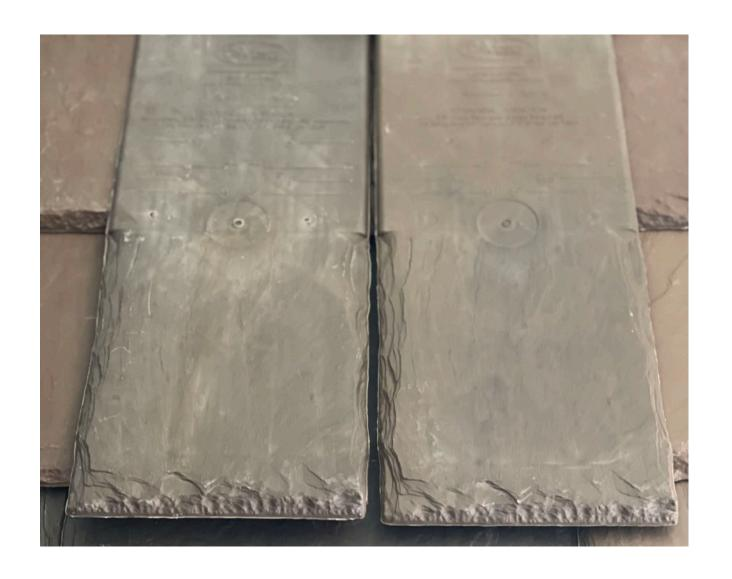
Raise the butt end of the overlapping tile(s) and place fasteners in the newly placed tile. The fasteners should be placed in the fastener placement circles along the sides of the tile or slightly below them. They should always be placed a minimum of ½" above the butt end of the course above and inline vertically with a nail placement circle.
