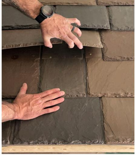
Place a new ring shanked nail or pancake head screw of appropriate length in each of the original holes where fasteners were removed from the upper overlapping tiles.
