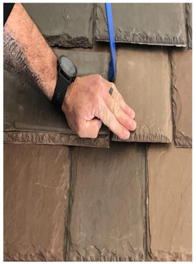
Press formed tile(s) flat to complete repair. Tiles may not lay completely flat immediately but should relax with warmer temperatures and time as long as the fasteners in the tile(s) are not over driven.
